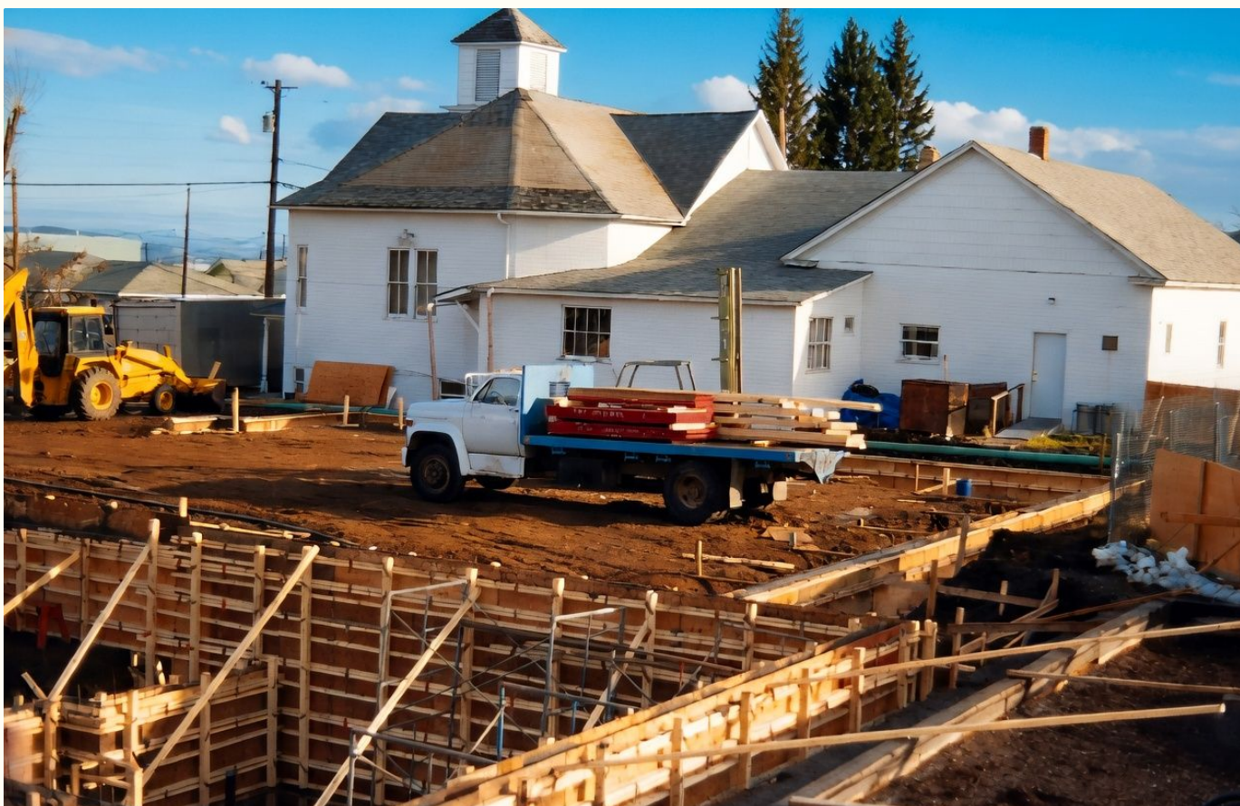
Phase One construction (archive photograph).
